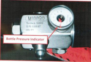
The firing head is installed on top of the bottle. The model of head used is a Mirada 5000. It will have a Serial Number and a Manufacture date.
